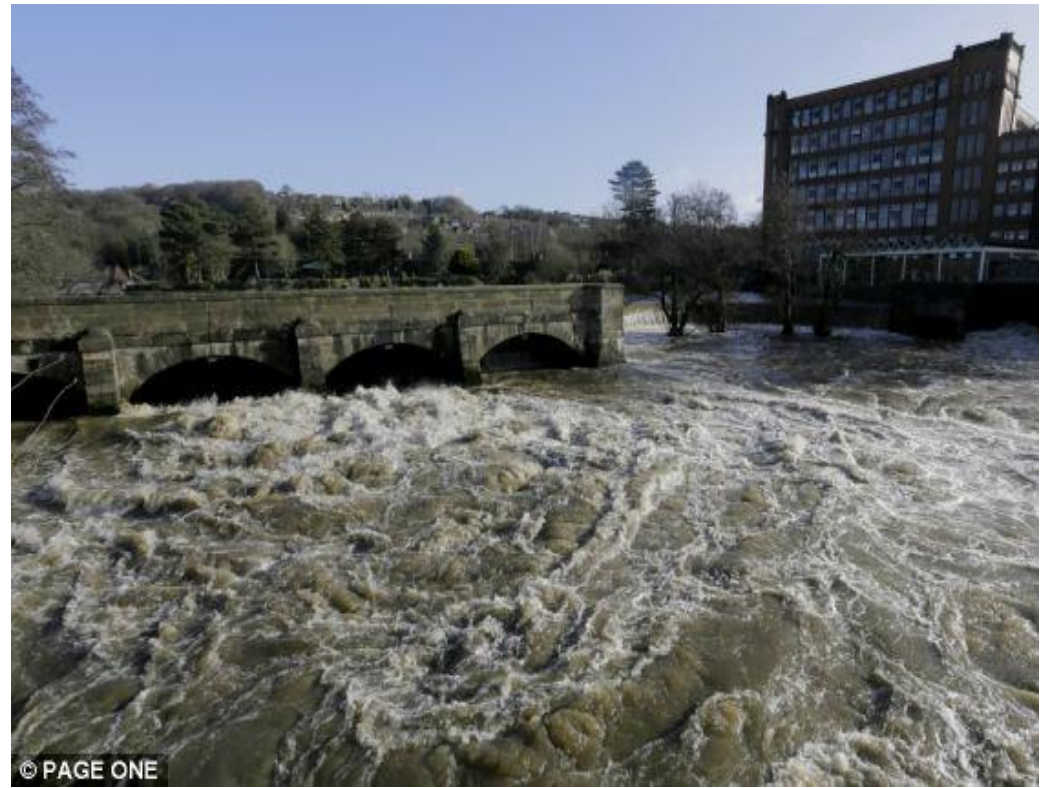
The river Derwent in flood in Belper (Jan 2013)
