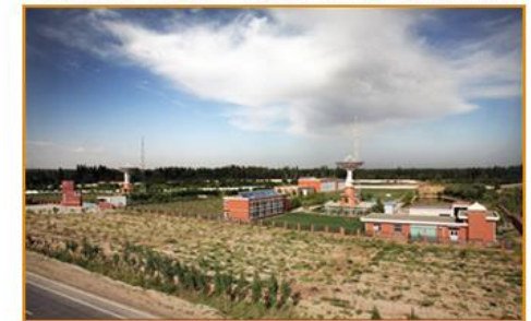
喀什站 Kashi Receiving Station
