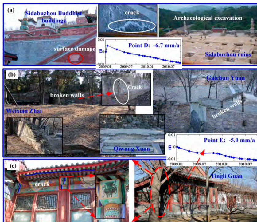
Figure 6. Photographs of Regions 2–4 marked in Figure 5a: (a) Region 2; (b) Region 3; and (c) Region 4. Displacement evolution of Points D and E (see Figure 5a for their locations) are illustrated by two sub-graphs.
